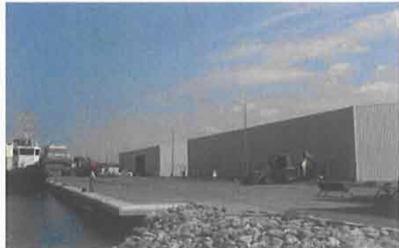
Installation of perimeter fencing surrounding the warehouse in March 2016
